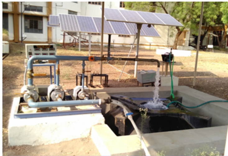
Solar PV Direct Drive Irrigation Pump (2015)
